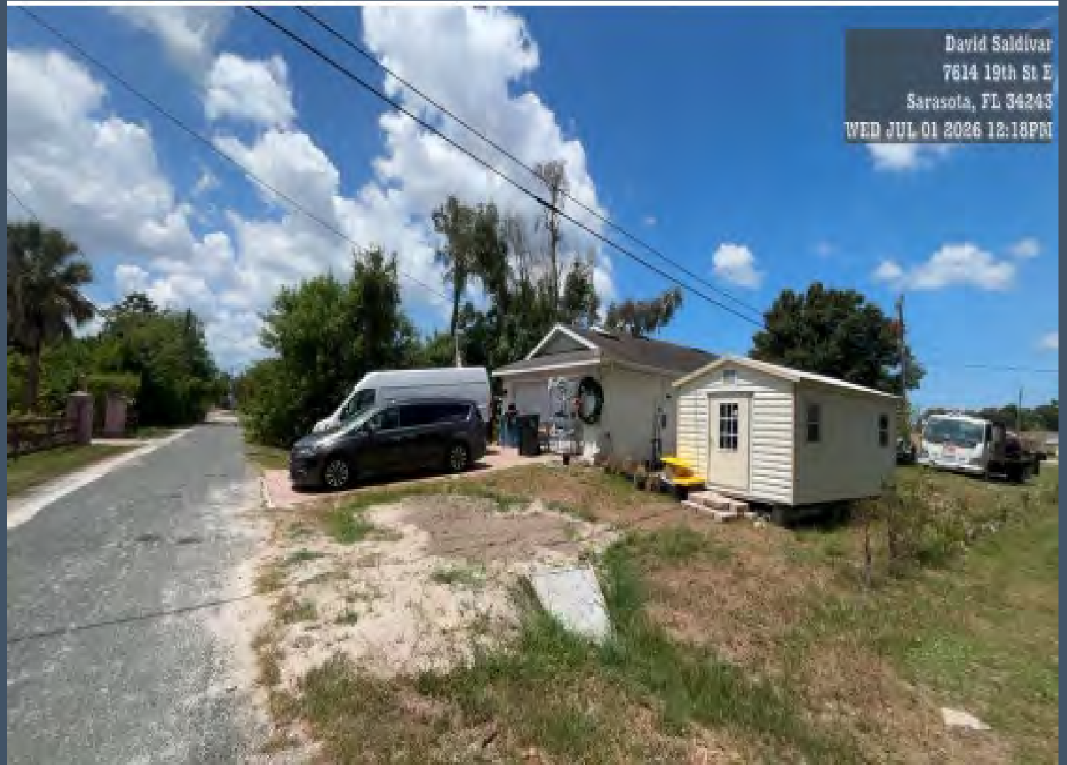
Picture depicts the unpermitted structure still on the property.
