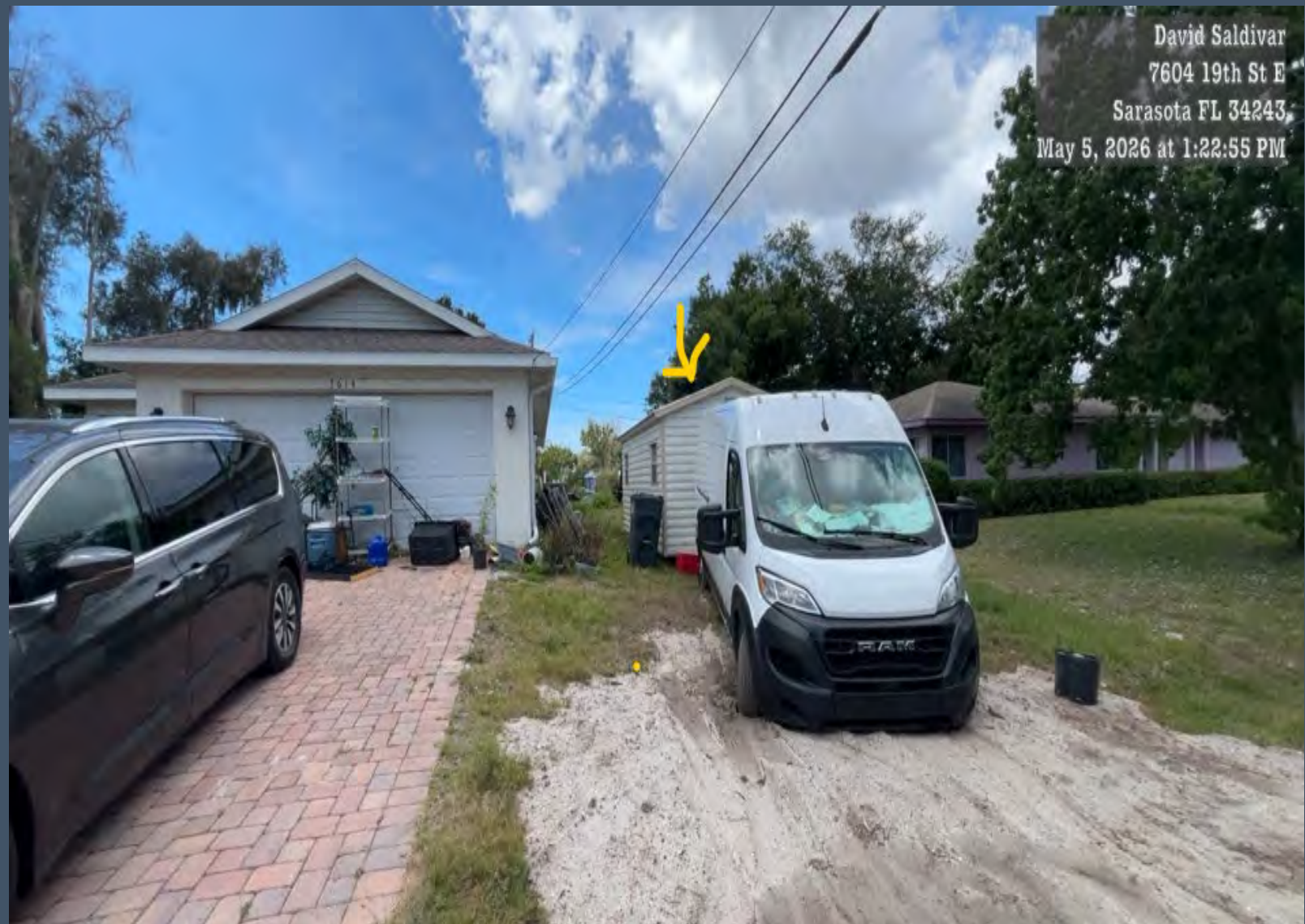
Picture depicts the front of the property and the unpermitted structure.
