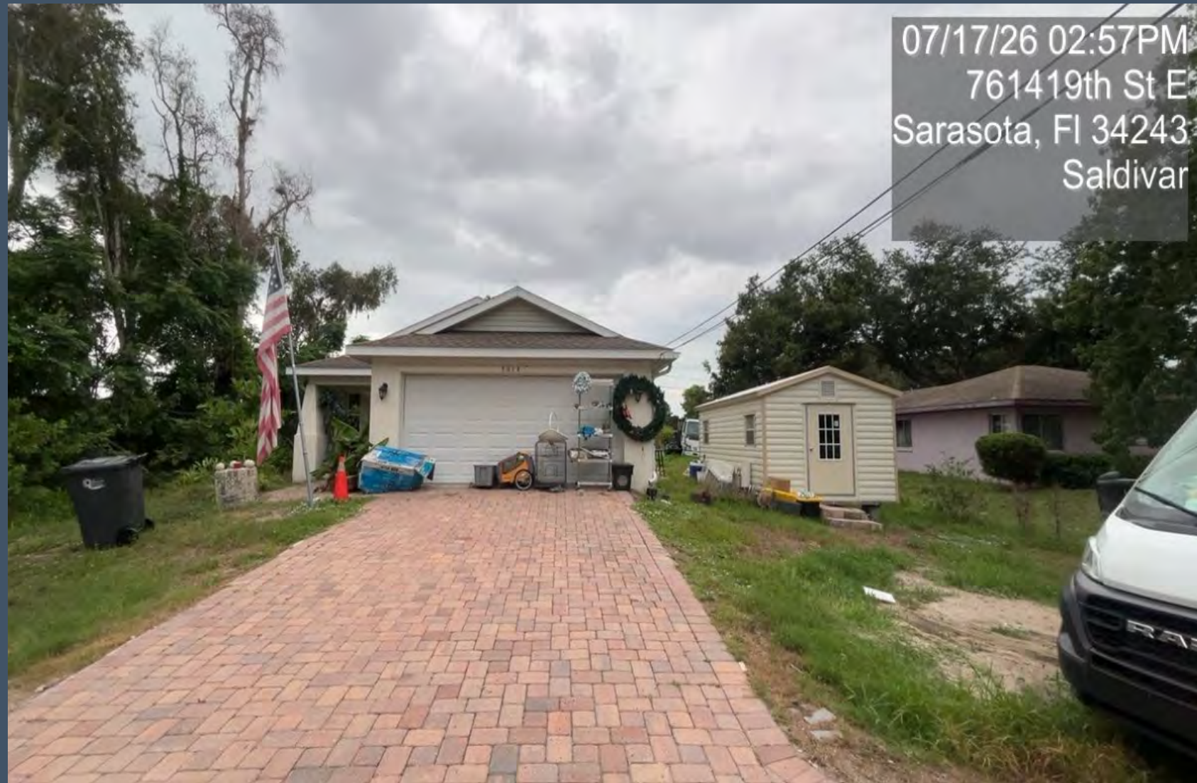
Picture depicts the front of the property and the unpermitted structure.
